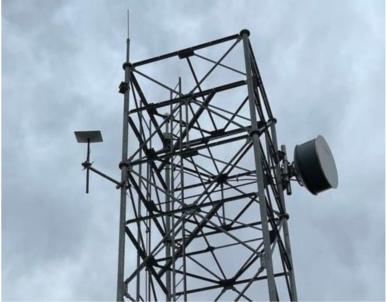
Figure 2.14: Starlink Ground Pole after installation at the Redding Fiber Hub
