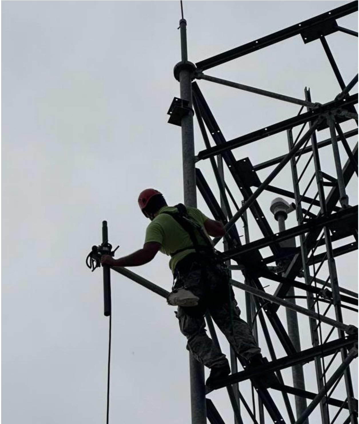
Figure 2.13: Starlink Ground Pole being installed at the Redding Fiber Hub
